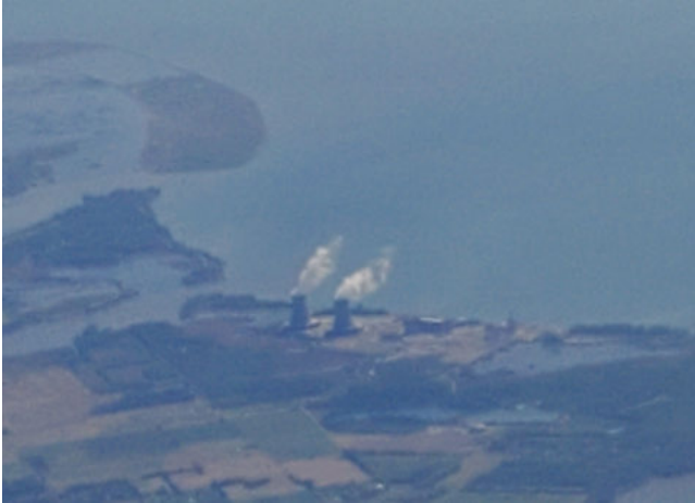
Figure 1.3: Aerial view of a nuclear power plant.
