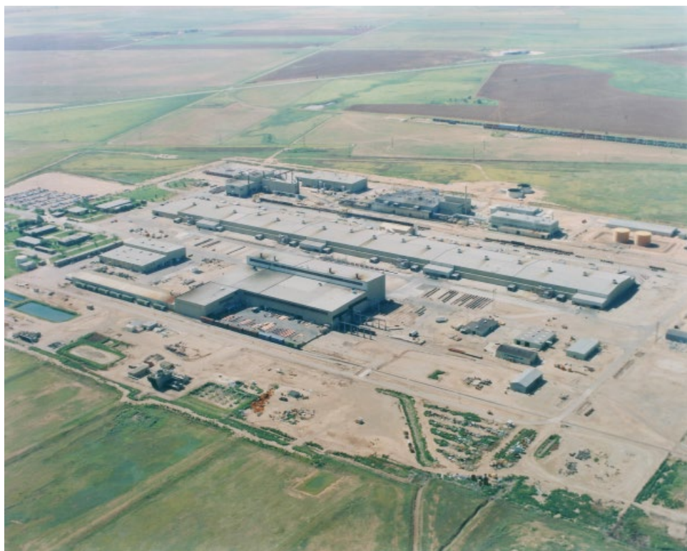
Figure 1 GV Asarco's Amarillo Copper Refinery (ACR) Tankhouse in Amarillo, Texas
