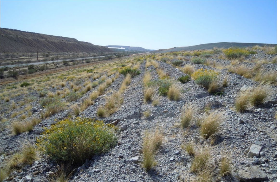
Figure 10 Revegetation success: side slopes of TSF in year 3. (See insert for color representation of the figure.)
