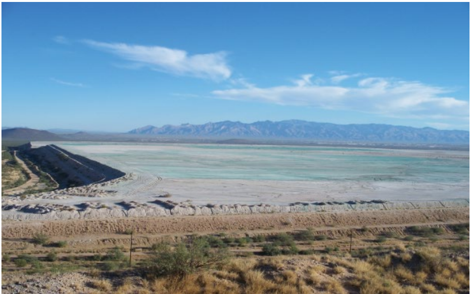
Figure 7 TSF before reclamation
