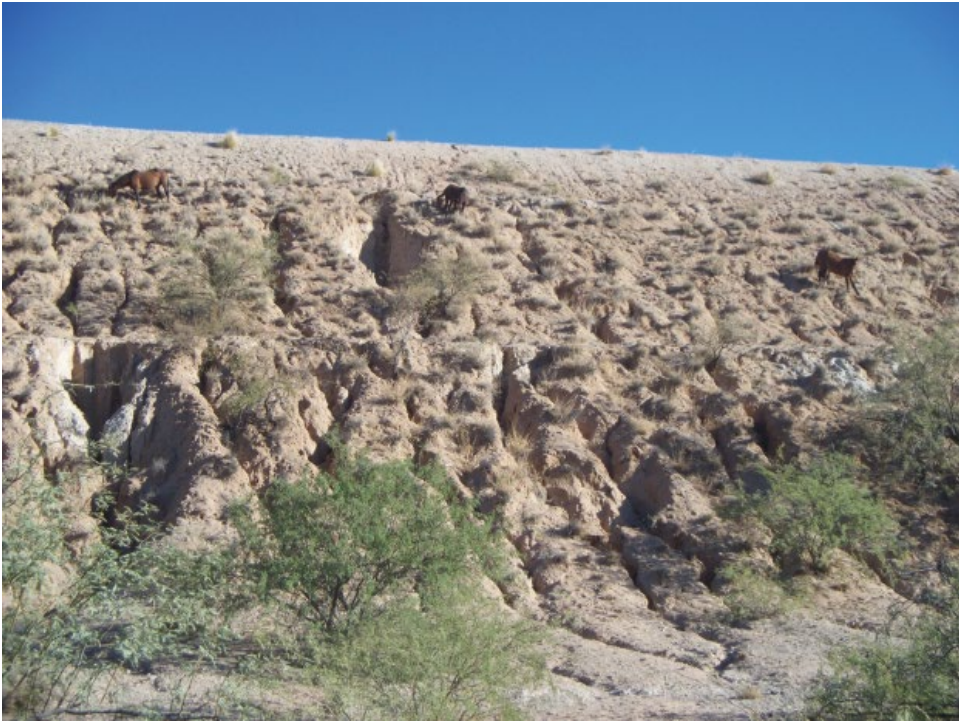
Figure 8 Benches and side slopes before reclamation
