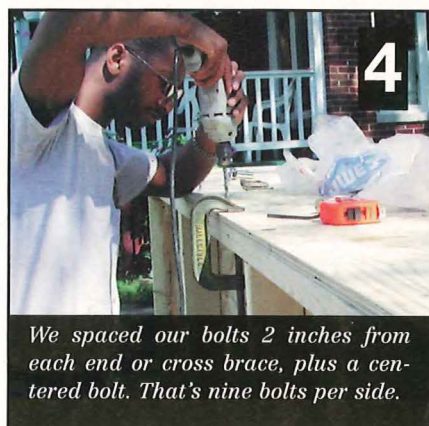
We clamped plywood to the frame, then worked our way down the 2x4, drilling holes and attaching bolts.
