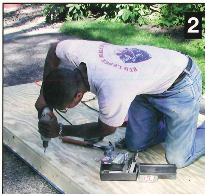
2 Brooks drives the deck screws slightly below the wood's surface to prevent cutting the liner. Before laying the liner, cover each screw head with duct tape or silicone sealant.
