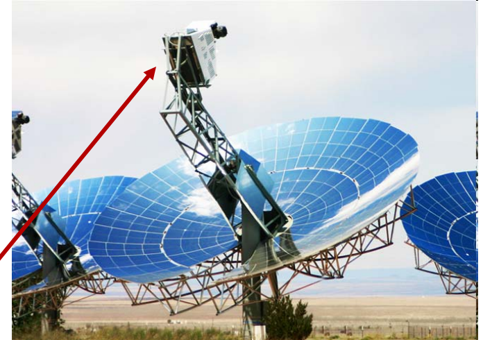
Tessera 20 kW Stirling concentrator dish
