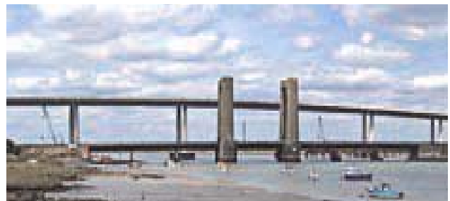
The Kingsferry and A249 Bridges
