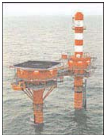
Oostdyck Radar Tower
