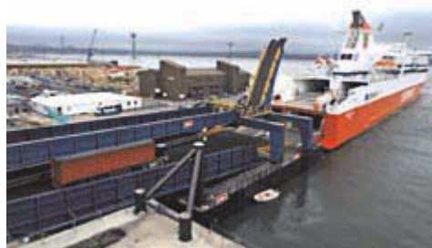
Rosyth Ferry Terminal
