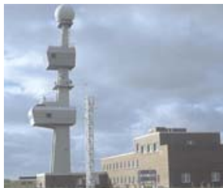
Knock Radar Tower (Light)
