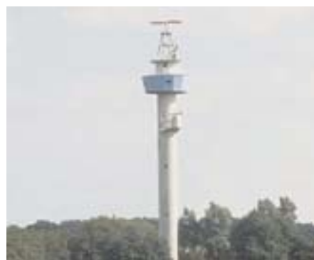
Tossens Radar Tower
