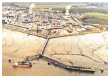
Salt End Oil Terminal
