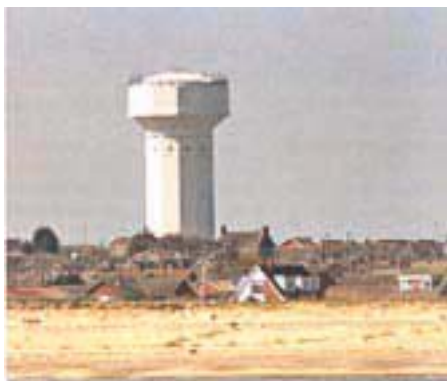
Caister water tower
