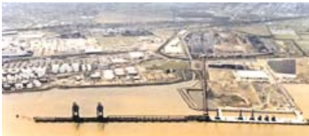
Immingham Bulk Terminal
