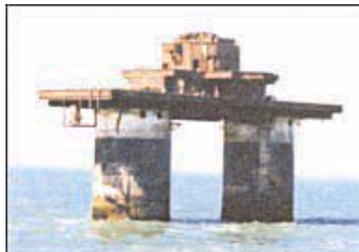
Knock John Tower
