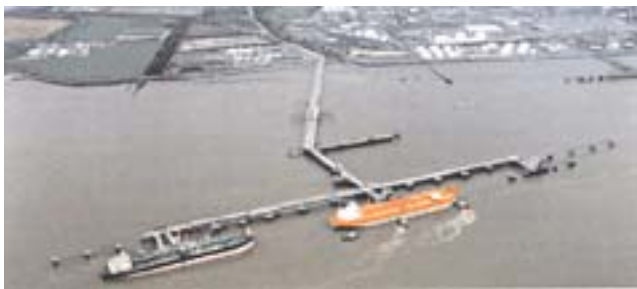
Immingham Oil Terminal
