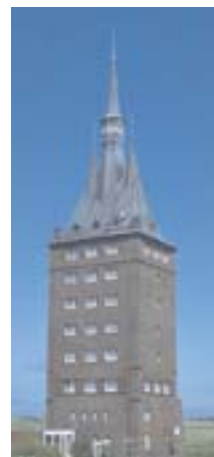
Wangerooge West Tower
