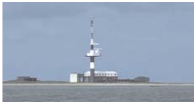
Oldoog Radar Tower (Minsener Oog Buhne C)
