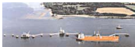
Hound Point Marine Terminal
