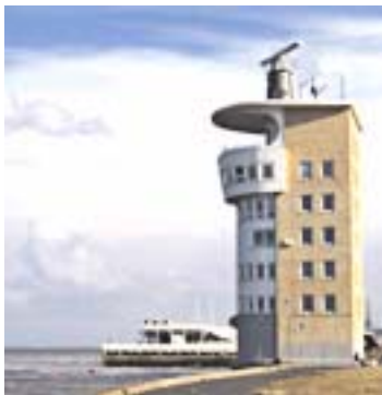
Cuxhaven Radar Tower
