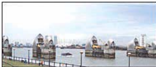
Thames Tidal Barrier
