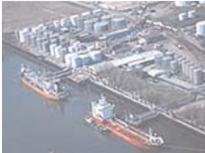
Hamburg Oil Terminal
