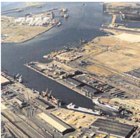
Tees Dock and Norsesea Oil Terminal
