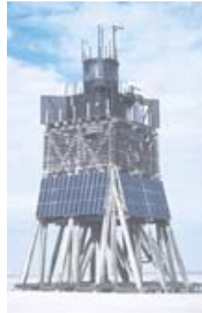
Suderoogsand Light (Refuge Beacon)
