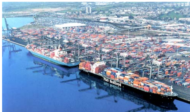
Southampton Container Terminal
