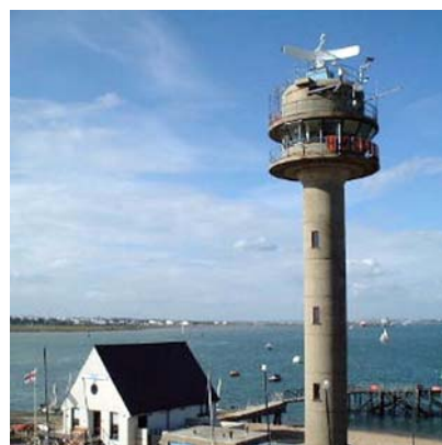
Calshot Radar Tower
