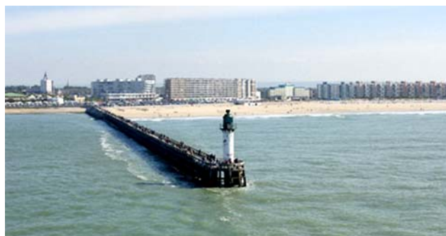
Calais West Jetty Light
