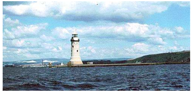
Plymouth Breakwater West Light
