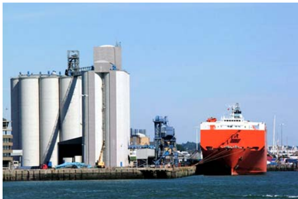
Eastern Docks Silo
