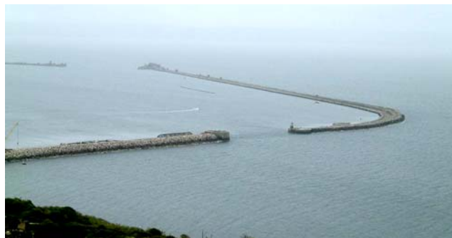
Portland Harbour Breakwaters
