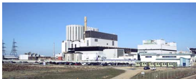
Dungeness Nuclear Power Station
