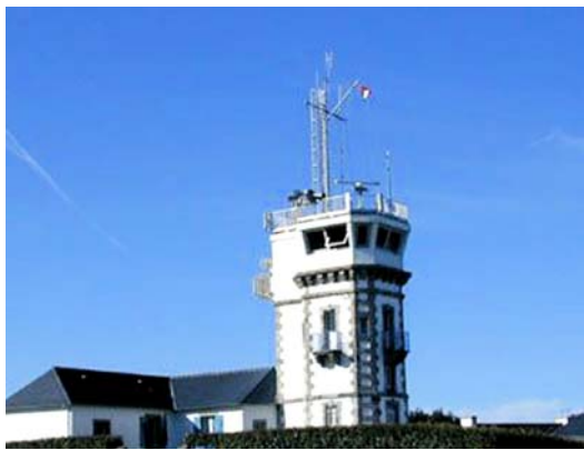
Ile de Brehat Signal Station
