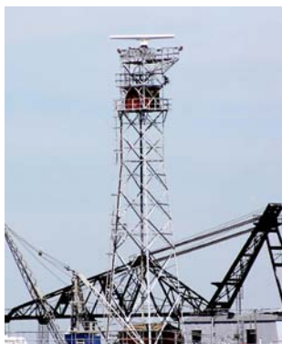
Admiralty Jetty Radar Tower
