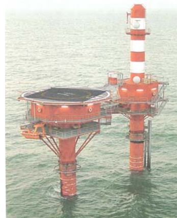
Oost Dyck Radar Tower
