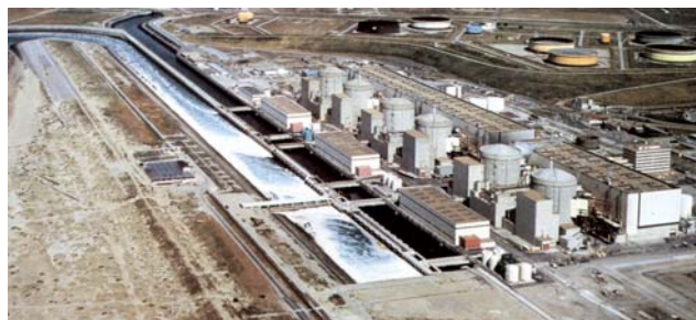
Gravelines Nuclear Power Station
