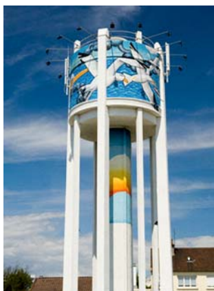
Calais—Bleriot-Plage water tower
