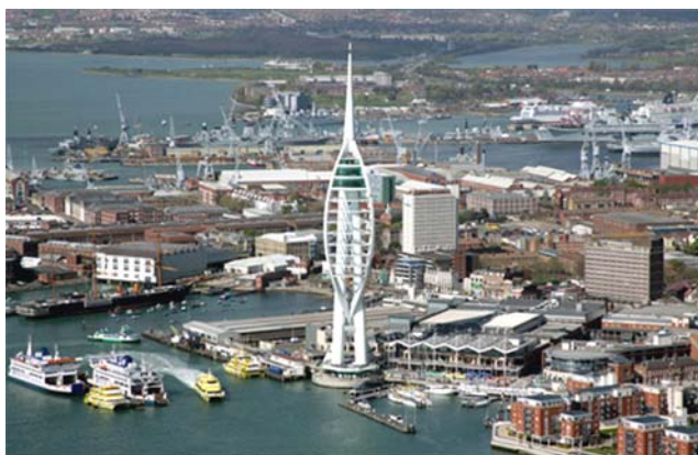
Portsmouth (Spinnaker Tower)
