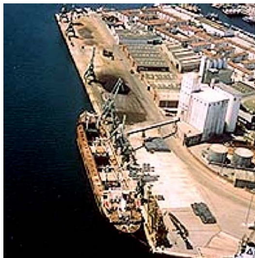
Santander—Margen Norte Quay (Maliano 1-7)
