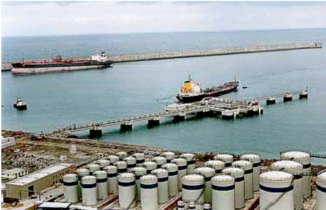
Bilbao—Punta Lucera Breakwater from SE
