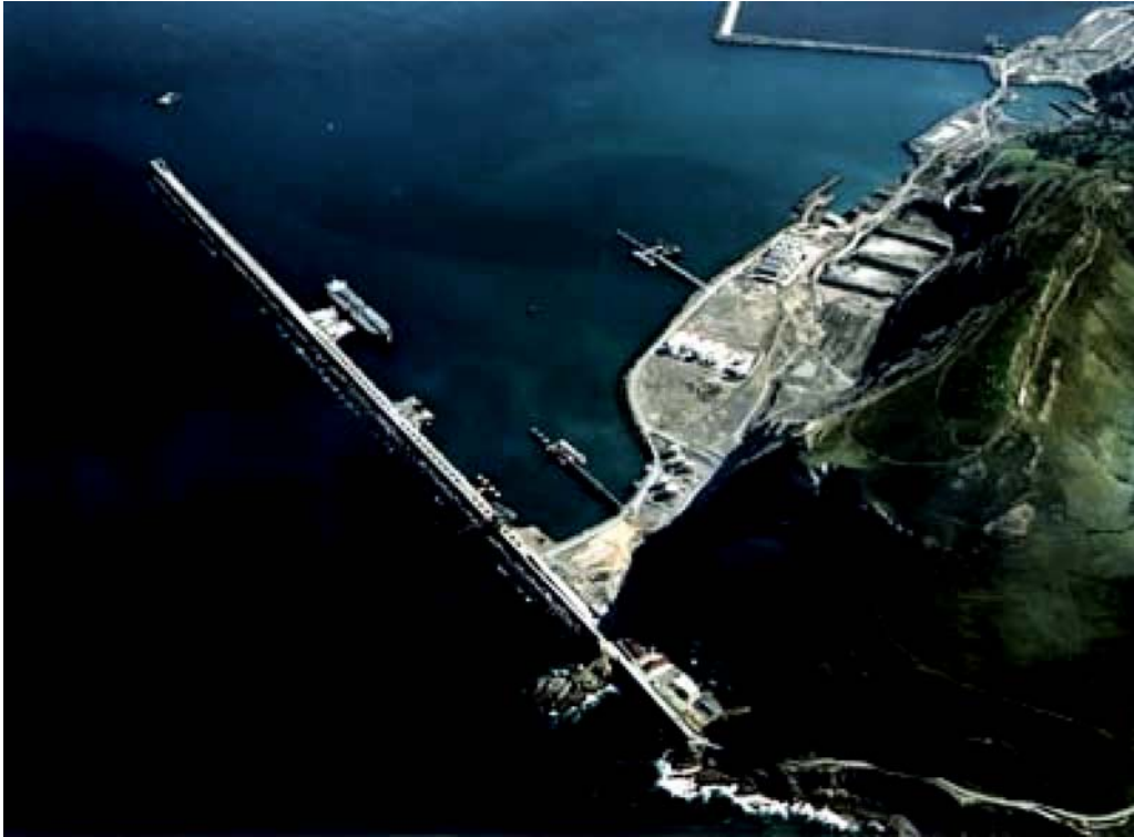
Bilbao—Punta Lucero Breakwater from W
