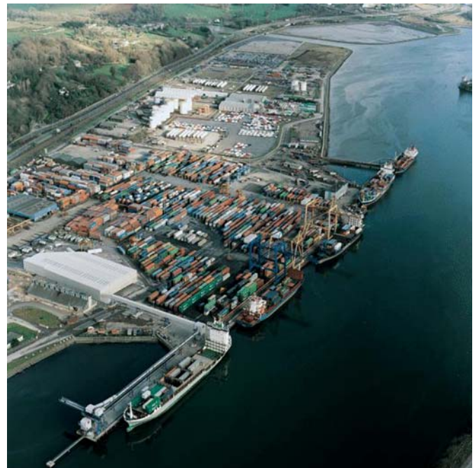
Cork—Tivoli Container Terminal
