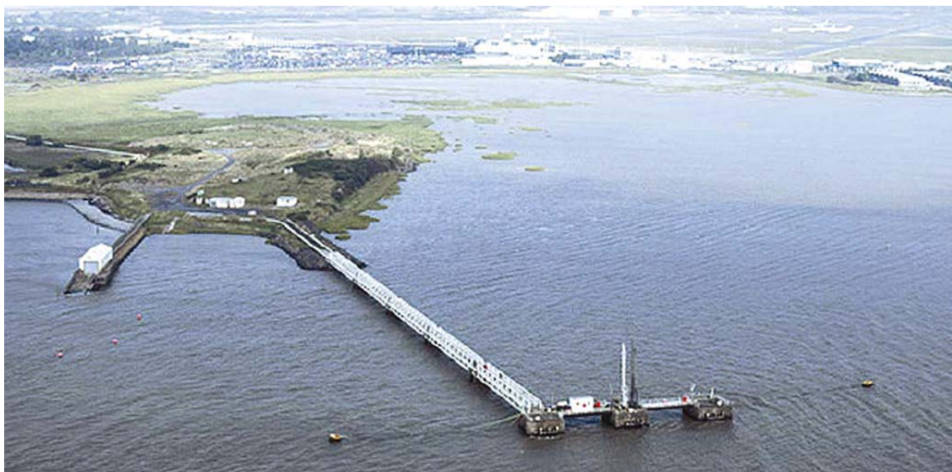
Shannon Airport Oil Jetty
