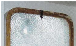
Further protection against flying glass can be provided by fitting security glass film
