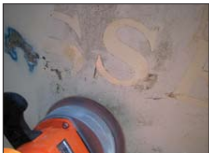
The 6" (152mm) orbital sander that I used for most of the project. The residue of the vinyl letters came off easily with the sander.
