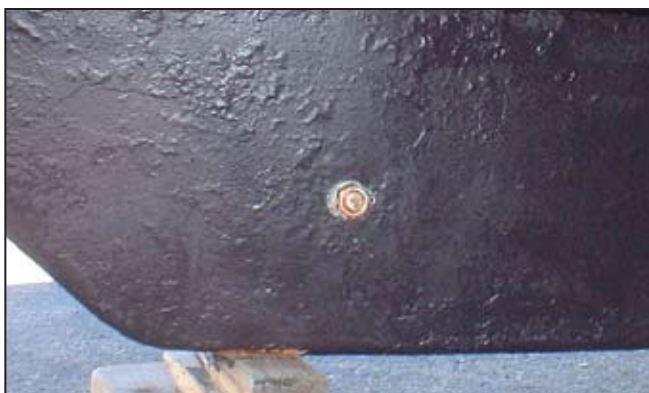
The finished job.
