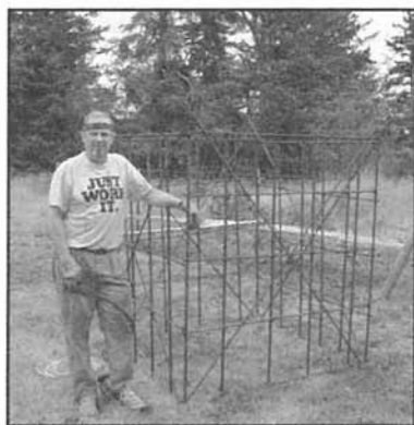
Photo 3: The finished cage after a couple of hours. Note the X bracing on each face. The extra lengths will be cut off with a hand grinder.
