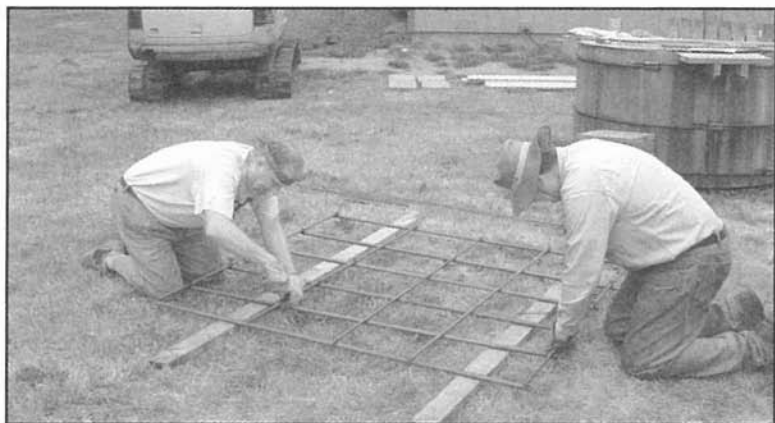
Photo 2: Building a rebar cage.
