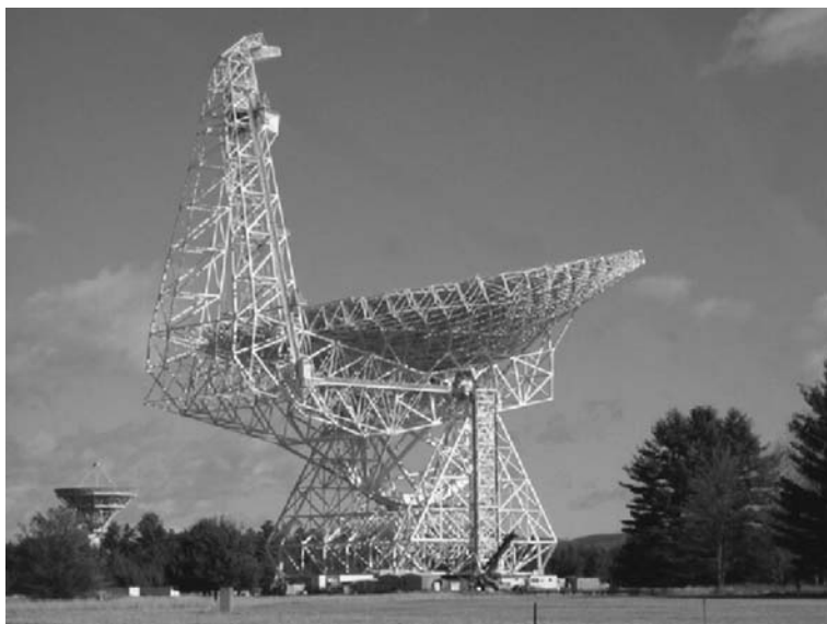
Fig. 7.11 The Green Bank Telescope (GBT) at West Virginia, U.S.A. The telescope is an off-axis paraboloid with a 110 m by 100 m diameter. This design was chosen in order to minimize side lobes and reflections in the telescope structure that lead to instrumental artefacts or “baseline ripples”
