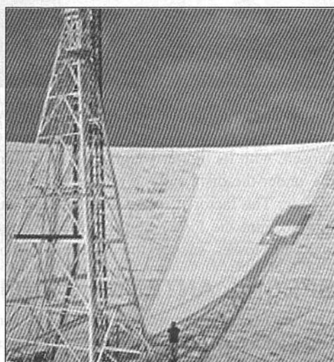
Fig 4.21: An early trial piece of the new galvanised surface. Note the thousands of mild steel plates laid during the Mk1A conversion. The ladder to gain access to the feed box is visible running up the tower. Note the size of the man standing at the base of the tower and the size of the low-loss coax cable. (Photograph by courtesy of University of Manchester Archives)
