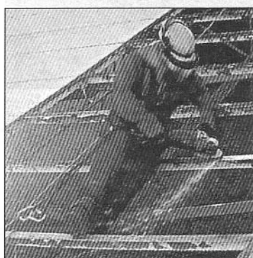
Fig 4.20: Grinding off the old welds after a section of panel had been removed. (Photograph by courtesy of University of Manchester Archives)
