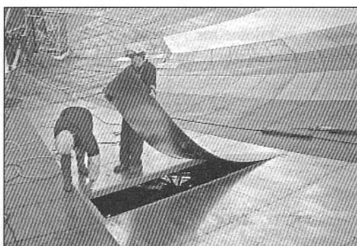
Fig 4.22: Fitting a new galvanised steel panel to the Jodrell Bank surface. The new panel has a bed of waterproof mastic to prevent corrosion. Note the many stainless steel screws fixing each segment in place. (Photo by courtesy of University of Manchester Archives)
