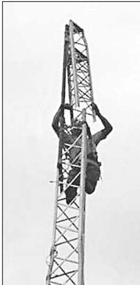
Figure 26.30 — Tower worker lowering a new section onto the top of the assembled stack of sections. The gin pole attached to the left leg is bearing the weight as the tower worker gives verbal instructions to the ground crew pulling on the haul rope. (Photo by Mike Hammer, N2VR)
