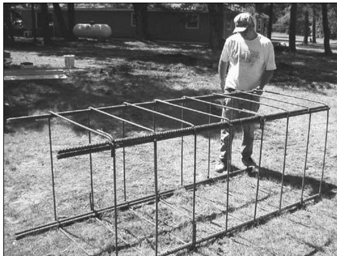
Figure 26.34 — The rebar cage for KX8D's tower base. (Photo by Duane Durlfänger, KX8D)
