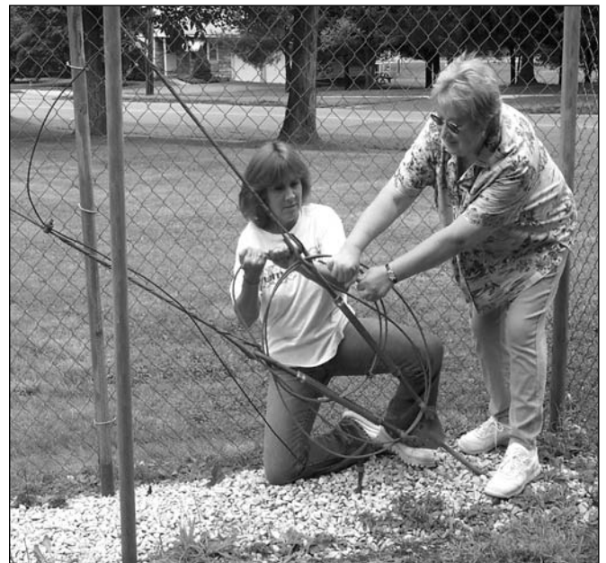
Figure 26.42 — A length of guy cable is used to assure that the turnbuckles do not loosen after they are tightened. This procedure is an absolute requirement in guyed tower systems, as shown by Jodi Morin, KA1JPA (left) and Helen Dalton, KB1HLF.
