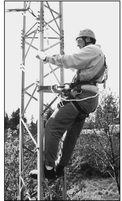
Figure 26.4 — A climber on a tower. Note the fall arrest lanyard attached to the tower above him.
