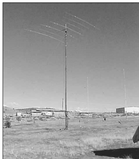
Figure 26.9 — Installation of surplus AB-577 tower with tribander at 45 feet at K7NV. (Photo by Kurt Andress, K7NV)
