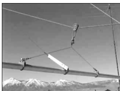
Figure 26.45 — Photo of the tram suspension system used by K7NV. Note that the tiller is attached to the haul rope in this system. The boom of the antenna can be rotated in the U-bolt holding it to the tiller to adjust the tilt of the elements to clear guy wires. (Photo by Kurt Andress, K7NV)
