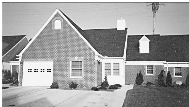
Figure 20.6 — The indoor loop is hidden inside at about the level of the dormer at right.
