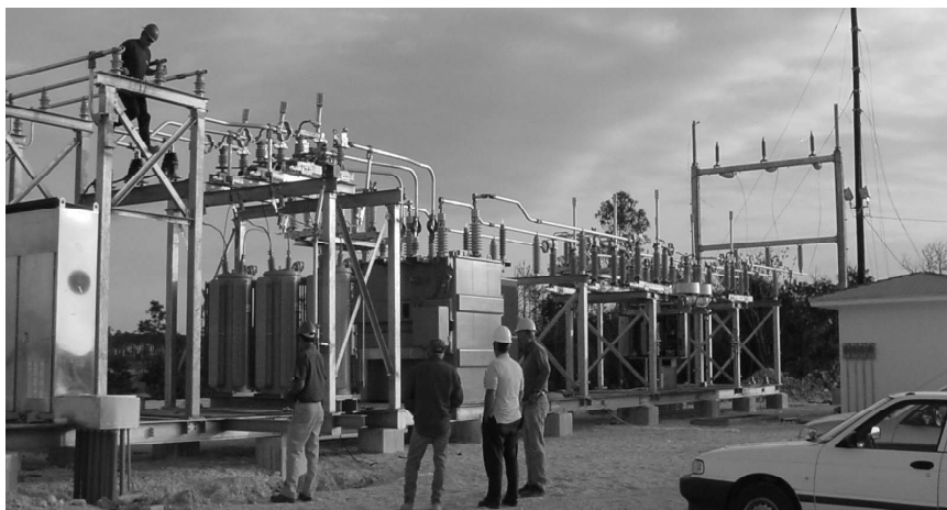
Figure 9.5 A nearly completed distribution substation under construction. Equipment in the foreground includes the distribution buswork and switching. In the middle is the transformer, and in the background to the left are the subtransmission switching and buswork. This particular substation is a modular design, built at a factory in several sections and trucked to the site, then assembled. Such substations require far less work than the traditional approach, which was to assemble all the components at the site.
