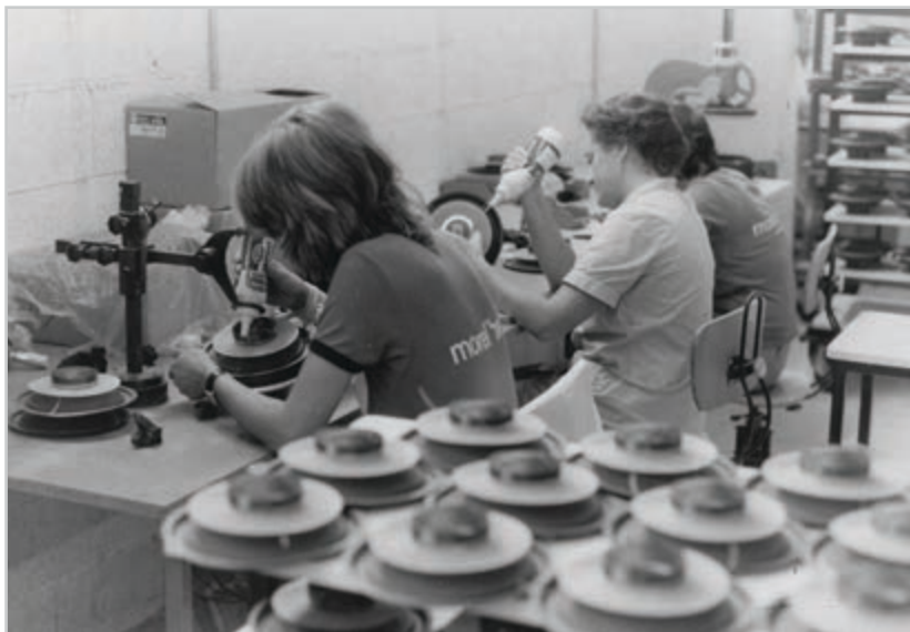
Morel's production floor workers are shown in this photo from 1980. (Photo courtesy of Morel)
