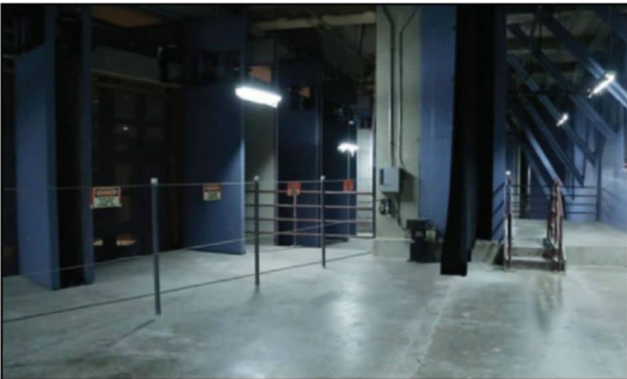
Photo 3: Mechanically operated curtains (look to the left of the stairsteps) covering a variable fraction of the reverb chamber's volume allow frequency voicing of the reverb character.
