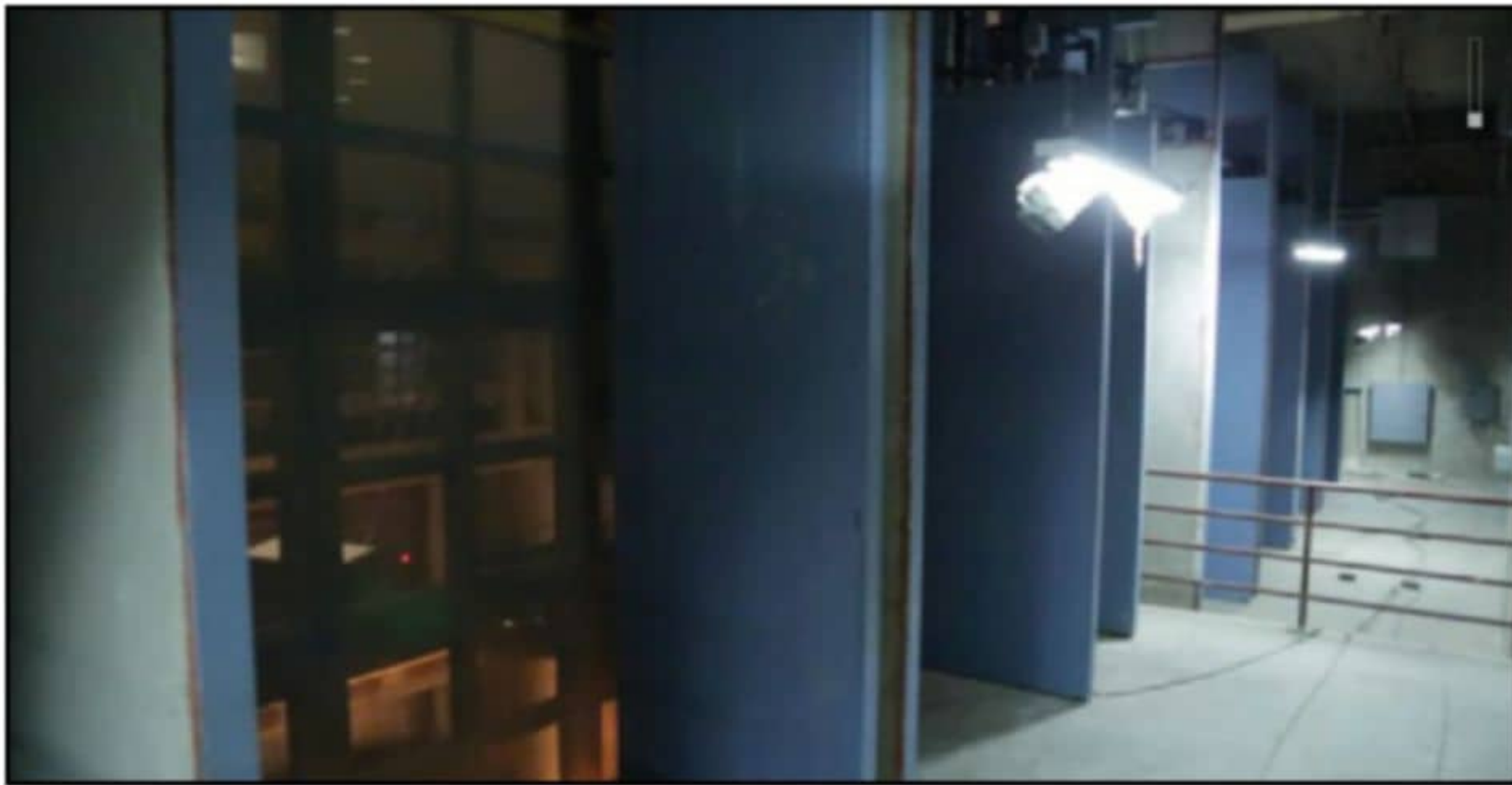
Photo 2: Mechanically operated doors control the acoustic coupling between the hall's volume and the reverb chamber.
