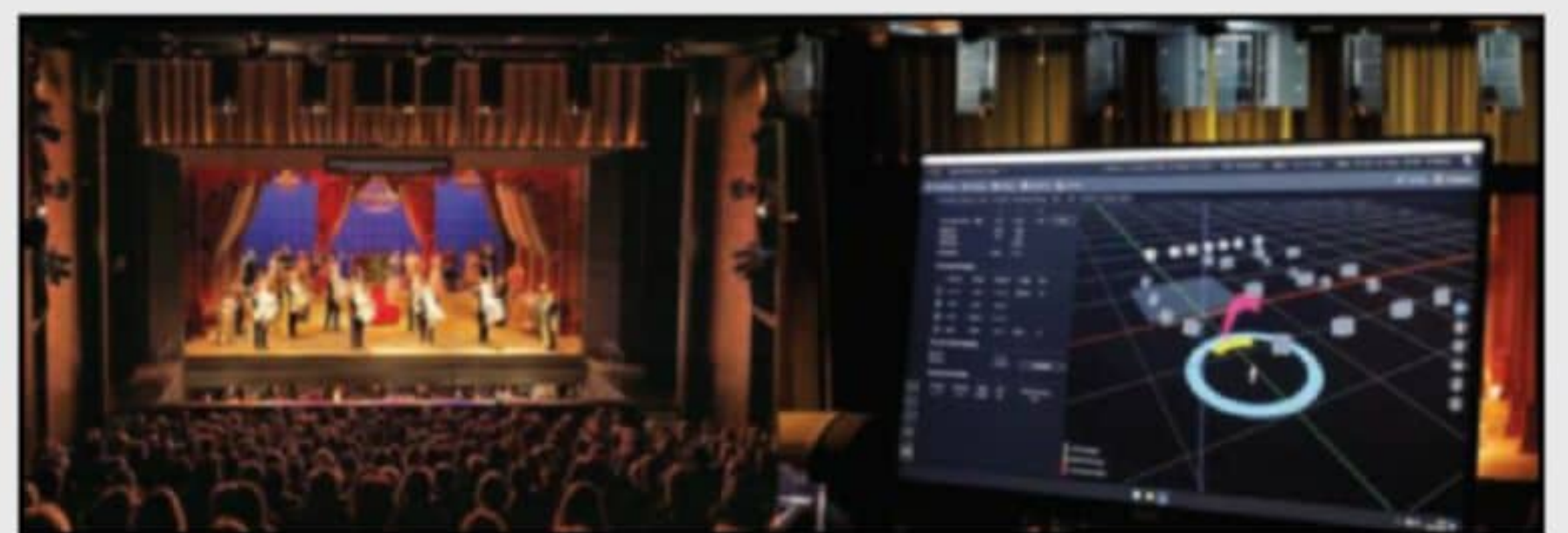
The first permanent L-Acoustics Ambiance Acoustic System was installed at The New Theatre, in Pulse, Czech Republic’s fourth largest city. With Ambiance, the room is now pre-tuned for orchestral music, operas, or theater productions, with a reverberation time from 0.95s up to 2.0s available with the simple press of a button on the L-ISA Controller.
