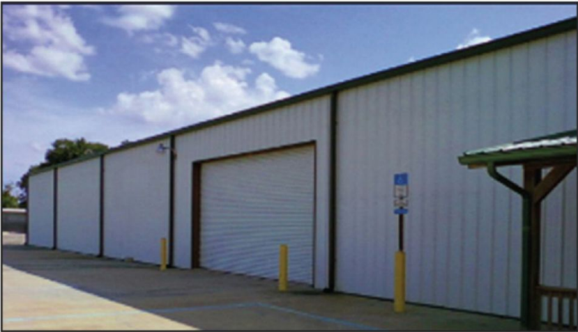
Photo 3: Using a commercial steel building can introduce acoustical design challenges.
