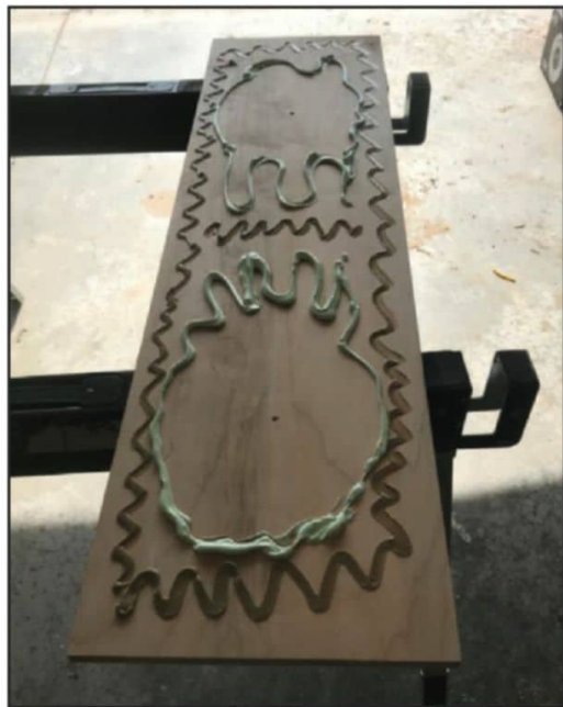
Photo 6: : I used Green Glue between 3/4" baffle layers. The Green Glue provides no-adhesion qualities, so construction adhesive is used to bond the panels near the perimeter and across the center.
