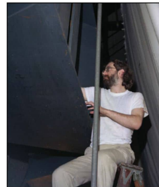
Taken in the 1970s, this photo shows the author hanging behind an Altec A-5 loudspeaker and suspended over a stage while changing diaphragms in situ. (Photo taken by Scott Norwood)
