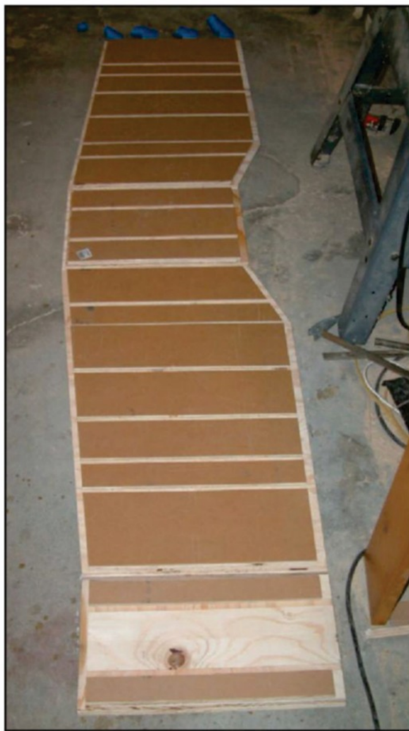
Photo 2: I laid the parts for the sides, top, and bottom of one speaker end to end.
