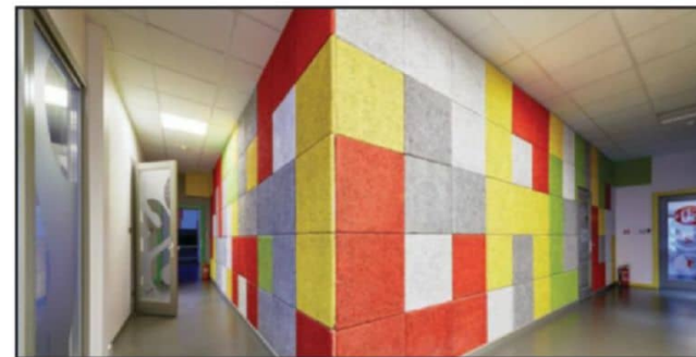
Envirocoustic Wood Wool panels can be mounted in ceilings or walls, are paintable and available with a wide range of SonoKote colors, and are an effective sound absorber.
