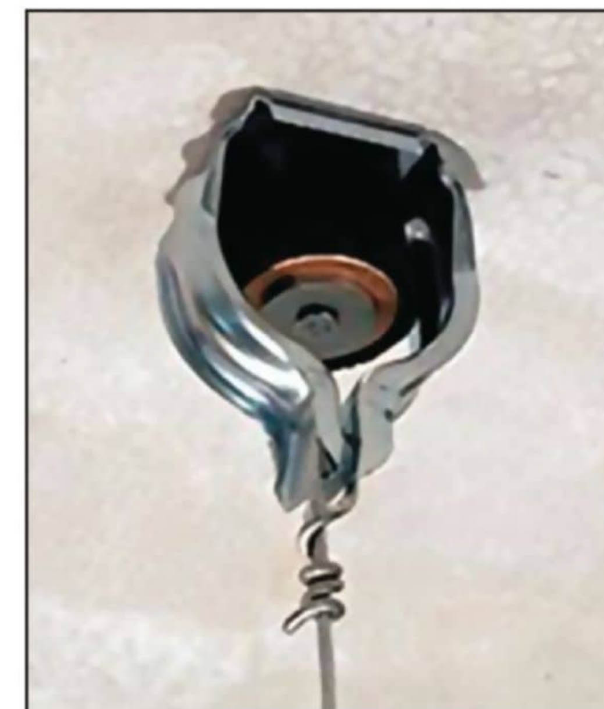
Photo 2: This resilient hanger can be used for a suspended ceiling.
