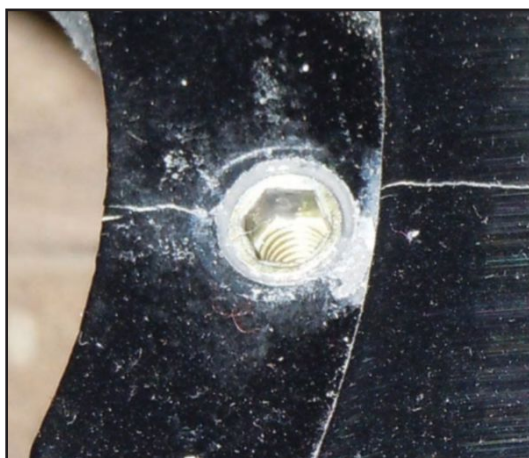
Photo 16: Installed EZ-Lok inserts
