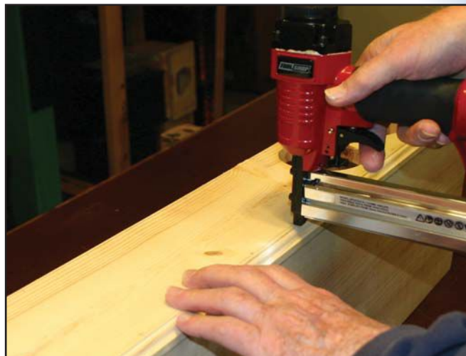
Photo 7: The enclosure can be assembled with finishing nails, a hammer, and a nail set tool, but the use of a pneumatic nail gun made the work faster and easier, with less risk of damage to the panels.
