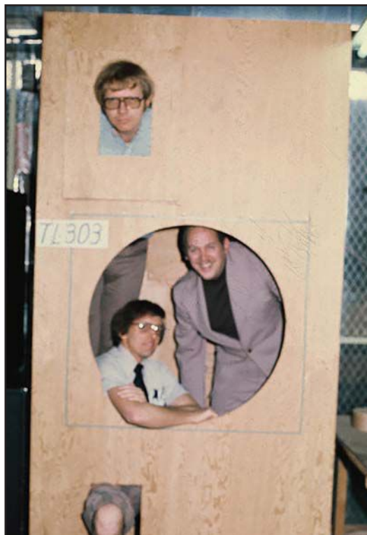
Photo 7: This is the large 76 ft 3 TL303 vented-box cabinet, which housed the EV 30W 30" driver. From top to bottom is Glen Meyer, Bill Raventos, and Don Keele. A speaker engineers' dream playhouse!
