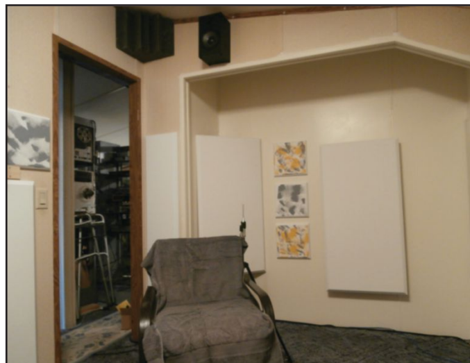
Photo 6 : This shows the alcove I created by removing a walk-in closet wall. One of the 2' x 4' panels is corner mounted and the other 2' x 4' panel is mounted 3.5" from the wall with special impalers. Both mountings provide bass trapping. Also shown is the right height speaker, part of the 7.1 setup, and three of my painted panels. (Perhaps I have a future in abstract art.)
