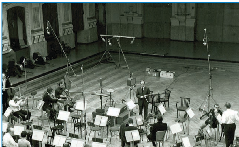
Photo 12: This is a Decca recording session in Vienna's Sofiensaal showing the Decca Tree in the center, above the conductor's podium. Decca invariably used the Tree along with accent microphones, but engineers have also used it as a purist, stand-alone configuration. (Photo courtesy of John Dunkerley, The Decca Record Co., Ltd.)
