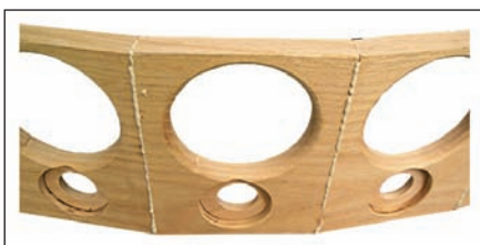
PHOTO 3: Polyurethane glue “fizz-out.”
