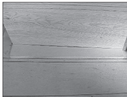
PHOTO 3: Checking brace for accuracy.
