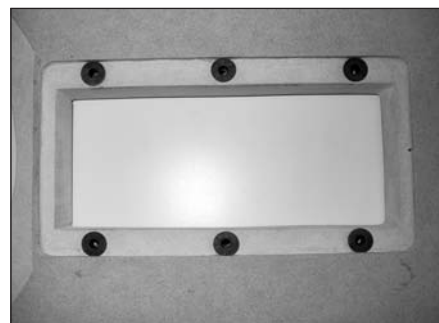
PHOTO 6: Rubber insulated rivet nuts.
