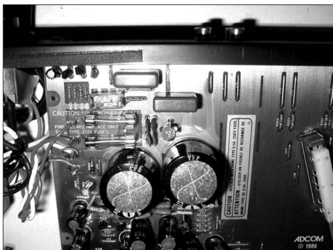
PHOTO 2: GFP-555 original power supply front.
