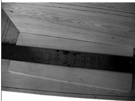
PHOTO 5: Dead-reckoning a brace.
