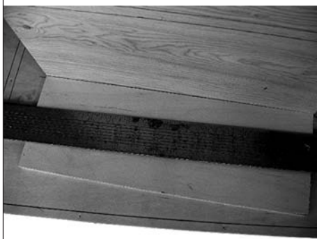
PHOTO 5: Dead-reckoning a brace.
