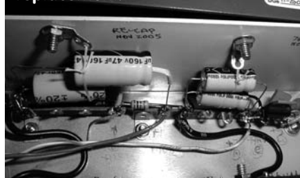
PHOTO 1: IG-4505 capacitor replacement.
