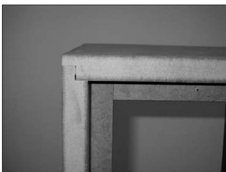
PHOTO 2: Panels L joints.
