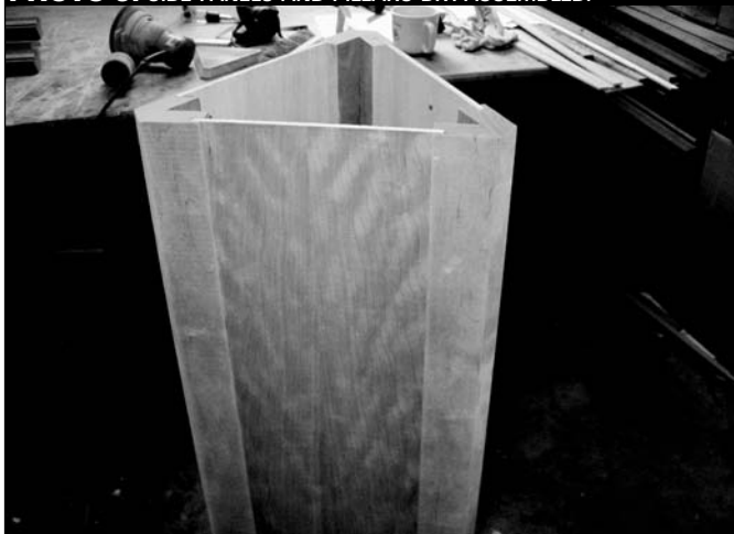
PHOTO 5: SIDE PANELS AND PILLARS DRY-ASSEMBLED.
