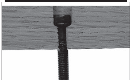
PHOTO 6: Cutaway of a counter-sunk baffle bolt hole.
