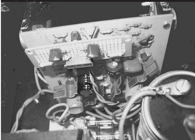
PHOTO 3: BALANCE BOARD INSTALLED.
