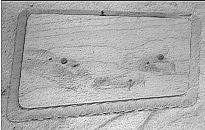
PHOTO 11: A FLANGED PORTHOLE COVER.
