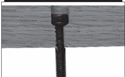
PHOTO 6: Cutaway of a counter-sunk baffle bolt hole.
