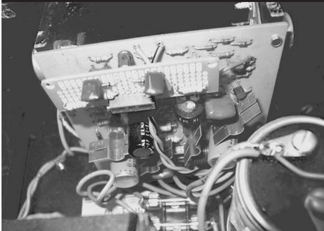
PHOTO 3: BALANCE BOARD INSTALLED.
