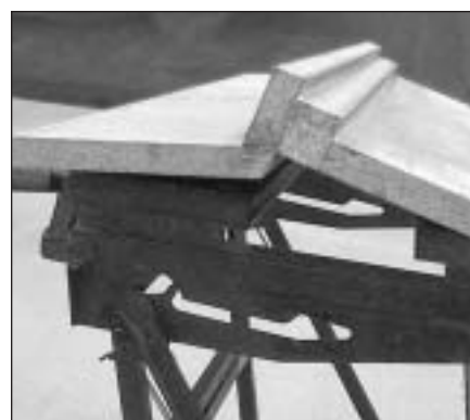
PHOTO 3: Assembling the bottom pieces.
