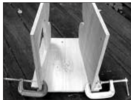
PHOTO 17: Using a jig to align the top and bottom for assembly.
