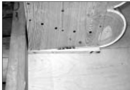
PHOTO 23: Rough-trimming the cabinet side.
