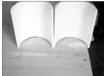
PHOTO 13: Tracing PVC halves onto cabinet top and bottom.
