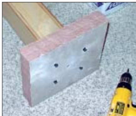
PHOTO 12: Attaching the sandstone base.
