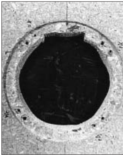
PHOTO 12: Front of hole to mount W3-871s driver.
