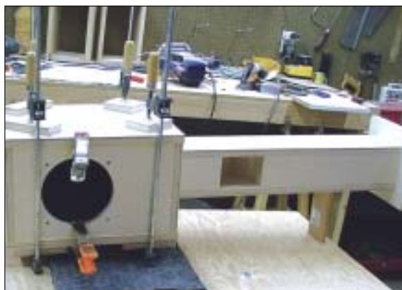
PHOTO 11: Gluing on the box sides.
