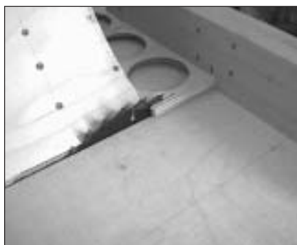
PHOTO 8: Trimming and squaring with the panel-cutting jig.
