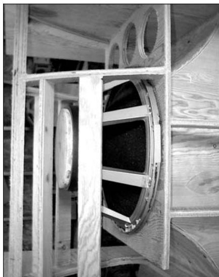
PHOTO 14: Make sure it fits! Note additional bracing.
