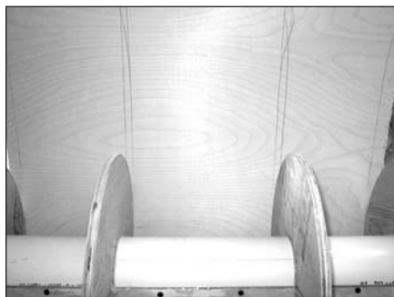
PHOTO 21: A back sheath marked for drilling pilots.
