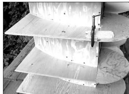
PHOTO 17: Using cauls to align a side brace.
