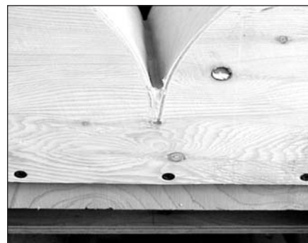
PHOTO 22: Filling the back sheath seam.
