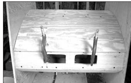
PHOTO 16: Attaching sheathing, step two.
