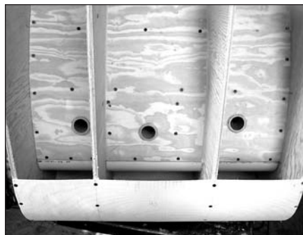
PHOTO 23: Location of the ducts.
