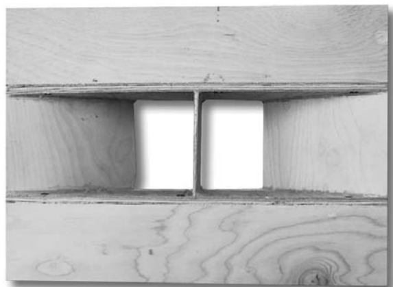
PHOTO 6: The throat horn attached to the horn supports.
