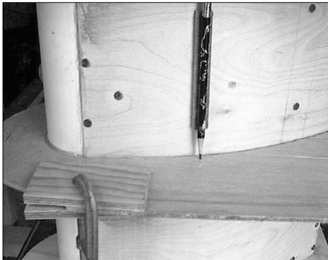
PHOTO 16: Attaching the side braces.
