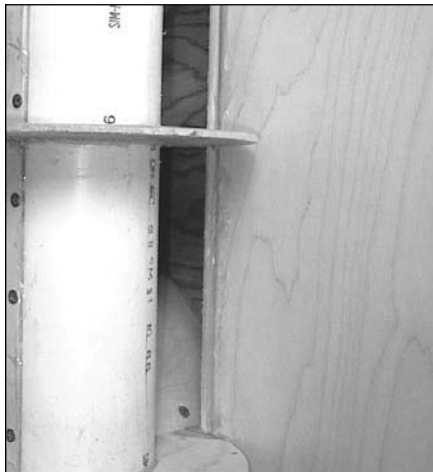
PHOTO 18: Beginning attachment of a back sheath.
