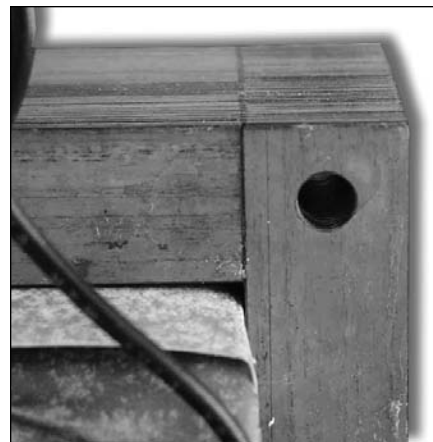
PHOTO 5: Close-up of the lamination gaps in an EI-core transformer.
