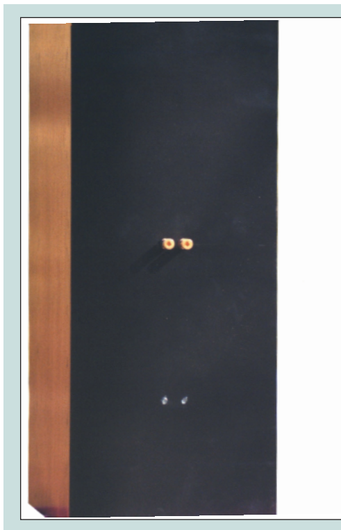
PHOTO 8: Binding posts have been moved to the center of the cabinet. Note pre-drilled holes when cabinets were built have been plugged with hot glue.
